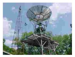
Squared Sqloop beacon antennas installed on one corner of the W4HHK dish platform.
